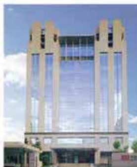
MEAN WELL GUANGZHOU TIANHE R&D CENTER
